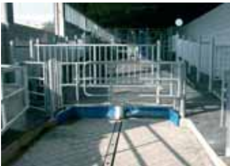
Divider gates and application of accessories on the passageways.
