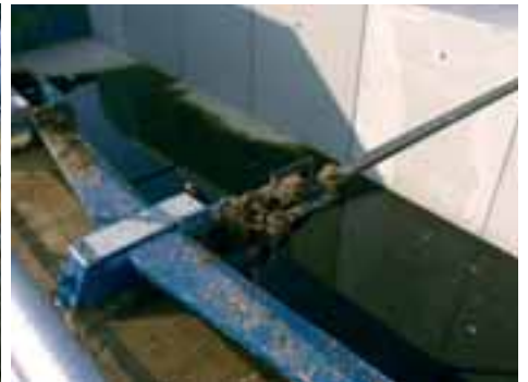
Flap scraper in the phase of discharge into tank.
