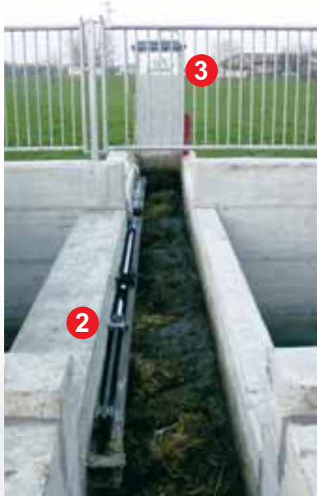
2 – Hydraulic unit for conveying towards the "Talpa" unit (3).
