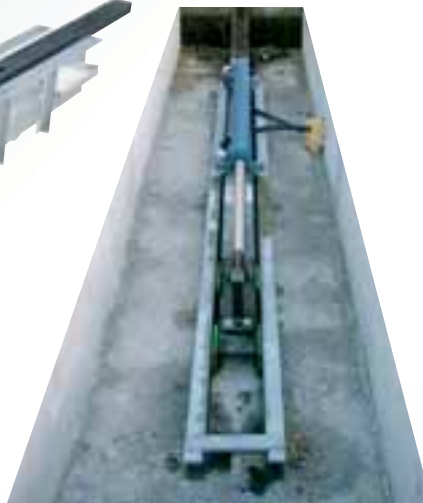
R.S.V. drive assembly with self-lubricating cylinder and guides in polyzene.
