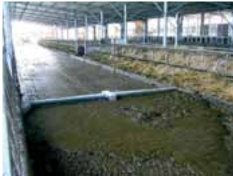
Flap scraper during cleaning.
