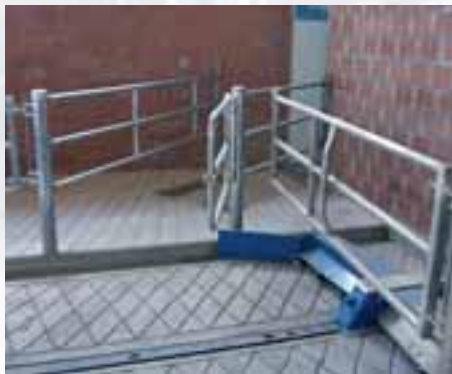
Detail of the return from the milking parlour
